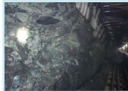
(a) Section of working face passing through cutting layer
