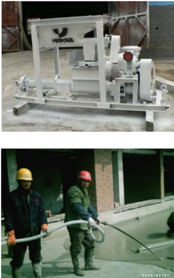
Fig. 7. Grouting pump and surface grout experiment
