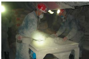
Fig. 9. Underground construction site
