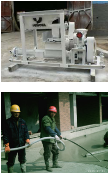
Fig. 7. Grouting pump and surface grout experiment
