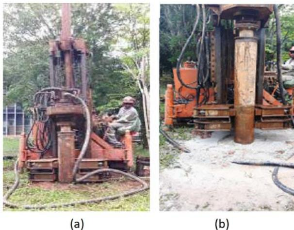
Fig.2. Construction of the energy pile: a) hydraulic drilling rig, and b) drilling process
