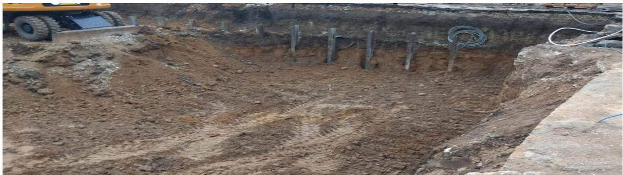
Fig. 2. Leveling of the piles.
